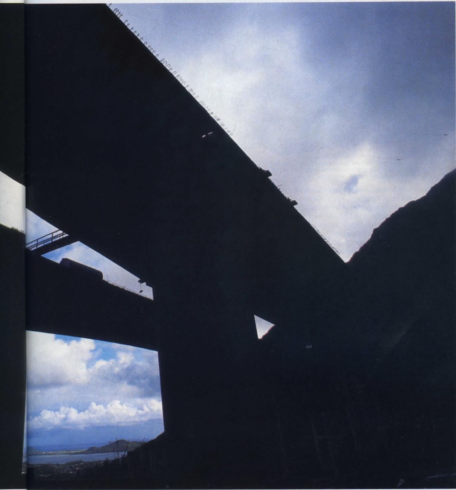
H-3 runs through Ha'ikū Valley on massive concrete piers, some higher than 100 feet.
