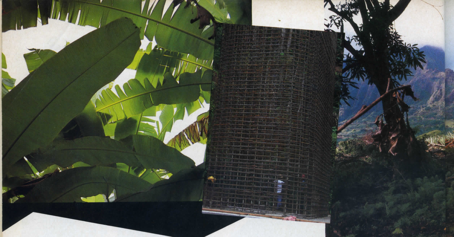
Above: A banana patch sprouting from ancient taro terraces—which were, until Hawaiian activists protested, slated to become an H-3 off-ramp. Above right: A forest of rebars grows to support an H-3 pier.
