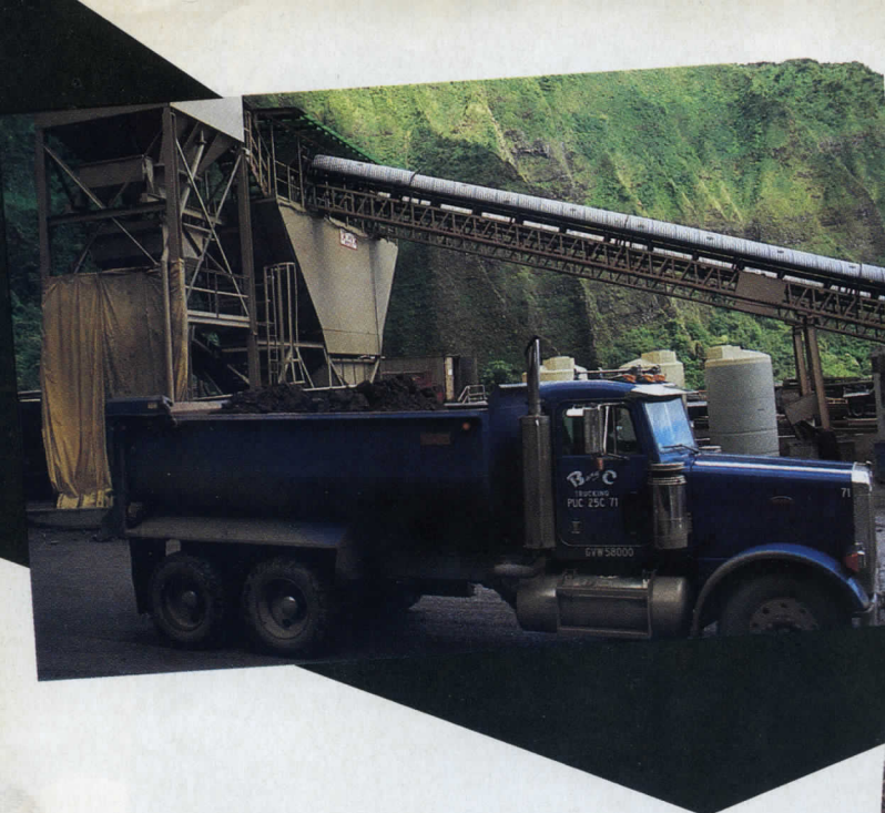
Above: A truck full of "muck" removed from the H-3 tunnels. Above right: The H-3 tunnels from the Ha'ikū end.
